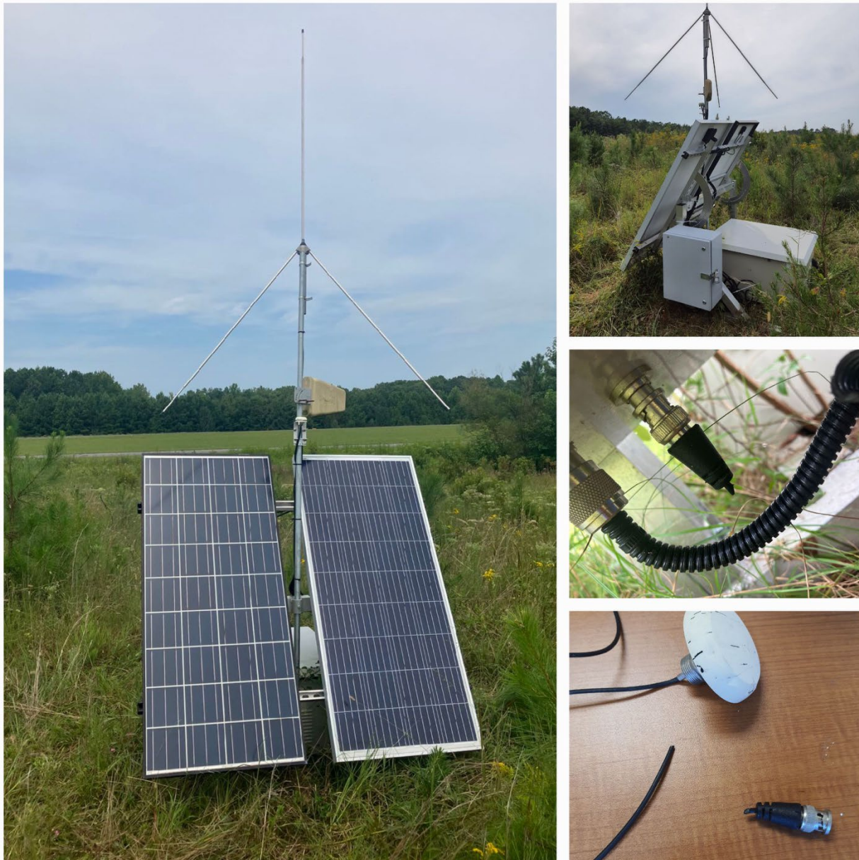
Figure 1. The Solar LMA and the damaged GPS coaxial cable at the UMD_UAS site.
