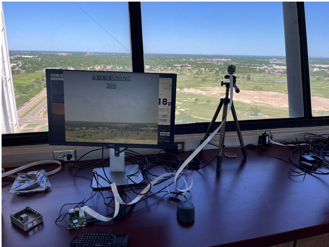
Figure: A new Raspberry Pi camera installed at Texas A&M University.
